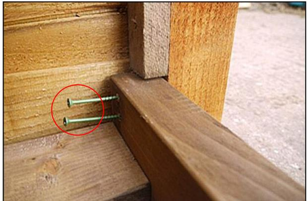
Attach the base to the end panel front posts using 2 of the 85mm screws for each side.
