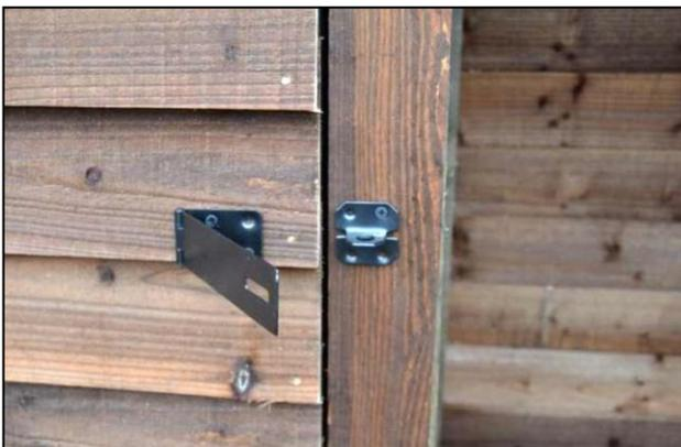
To fit the latch keeper plate, shut the door and hold the latch in the horizontal position. Now fit the keeper and mark its correct fixing position on the post using a pencil or bradawl before securing it in place using the screws provided.
