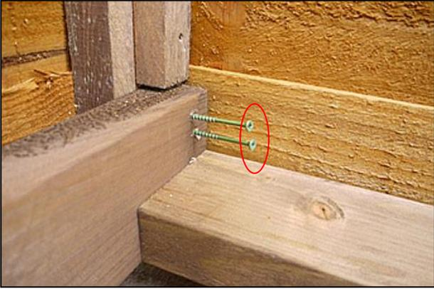
Now attach the base to the end panel rear posts, again using 2 of the 85mm screws for each side.
