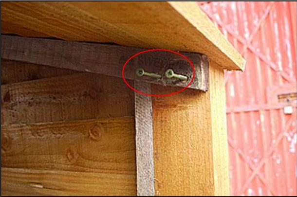
Check that the front batten ends sit flush with the posts as shown. Now attach the roof to each end panel post with 65mm screws.
