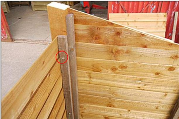
Secure the right side panel in place with 65mm screws.
