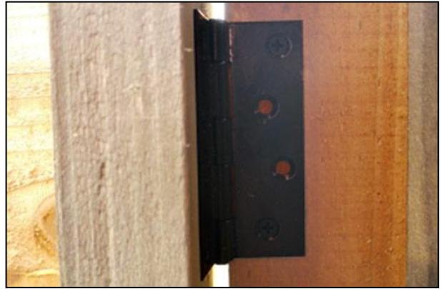
Align the top hinge in place, ensuring that the gap between the door and post is consistent at top and bottom then secure the top hinge in place using more of the black hinge screws
