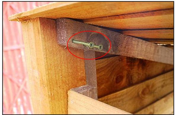
Secure the rear of the roof using 65mm screws as shown. Your log store is now complete. If your log store came with doors, proceed to step 13.
