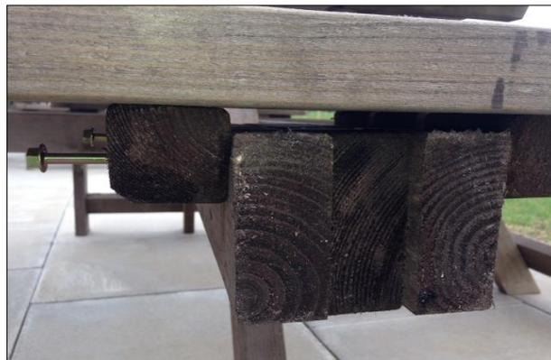
...noting the clearance between the seat and the upper surface of the frame assembly. Repeat steps 8 - 10 for the remaining seat units.
