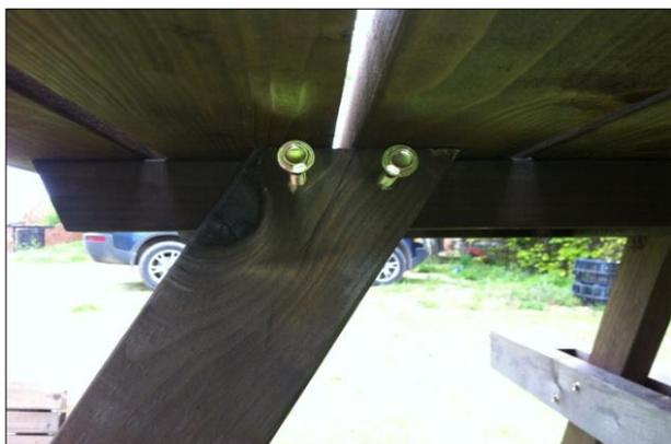
Now attach the table top to the leg assembly using 2 coach screws per leg.
