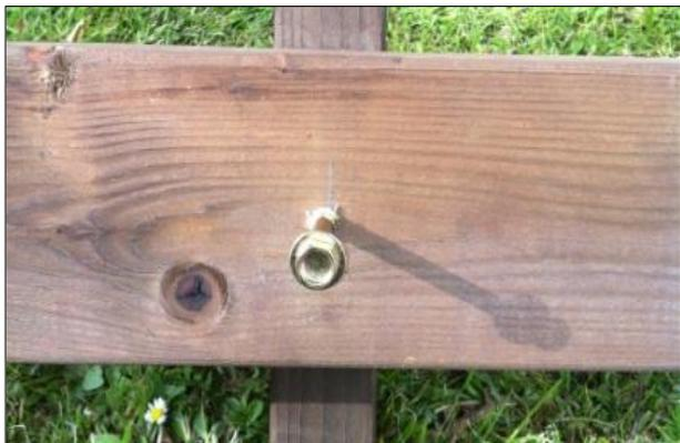
...and attach it to the leg using a coach screw...
